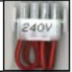
**NOTE:** Before making any electrical connections to the power supply, remove the access door panels, open the control box and check the correct plug (240 volt) is installed.
